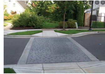
Strip of pcc blocks to slow traffic arriving on site
