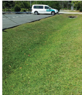
Shallow grass swales to act as bioretention to surface water runoff from roads
